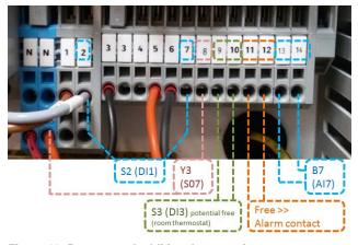
Figure 11: Prearranged additional connections C6.1.6/1017-1219/E
