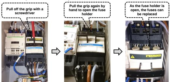
Figure 23: Replacement of the fuses
